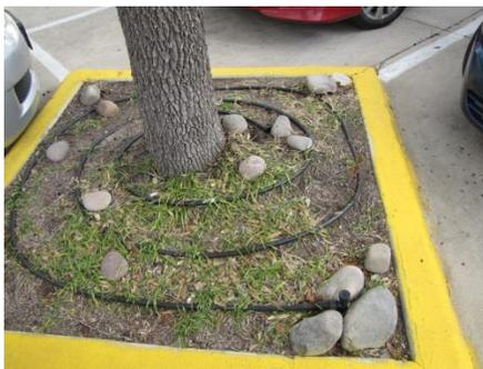
Drip Tubing Attached to Sprinkler
